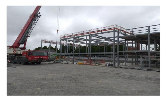
Last steels that form the superstructure being lifted in with the 100-ton crane, the edge protection for roofing works is fixed to the steel before it is lifted up to avoid the need to work at height
