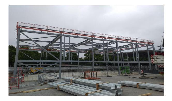
All steels lifted in and bolted together to form the completed superstructure
