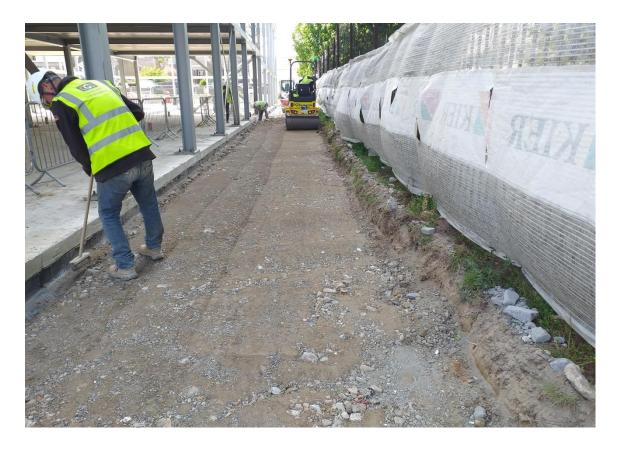
The 3-Metre-wide excavation around the whole building is filled with 300mm of crushed material and compacted down with the use of the roller to form a stable base for the scaffold and mobile access equipment
