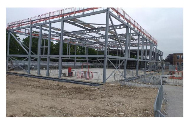
The cranes last lifts were to lift in the structural deck, you can see the packs loaded onto the roof ready for install
