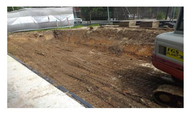
3-Metre-wide excavation around the whole building is dug away, this will be for the Scaffold and Mobile access equipment to go on so they can access the higher levels
