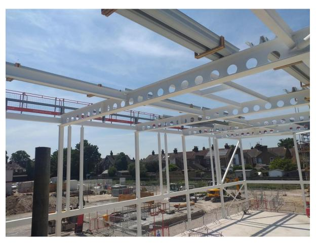
In this photo you can see the steel has changed colour from grey to white, this is a spray applied intumescent coating that gives the steel its fire resistance
