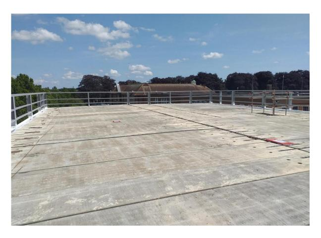
Roof of the teaching block, top of the structural planks ready for the structural topping
